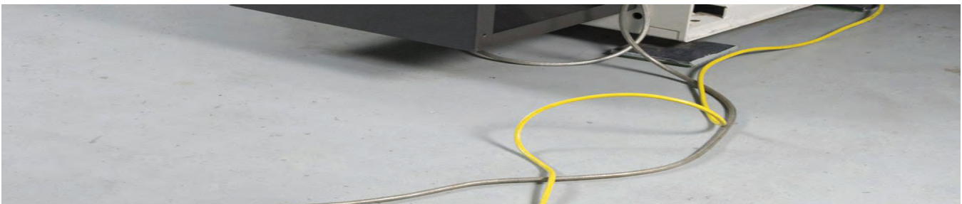
Image 4.1 – Loose cords and wires with lack of contrast with the flooring
